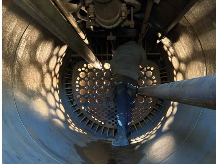
**Jack Harper trial fitting small and flue tubes.**
