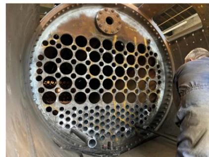
**The process of fitting the small tubes.**
