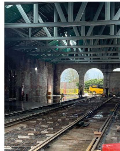
**Work in progress to restore the 1861 Whessoe Road engine shed, note the new roof trusses in place and preparations to pour the concrete floor.**
