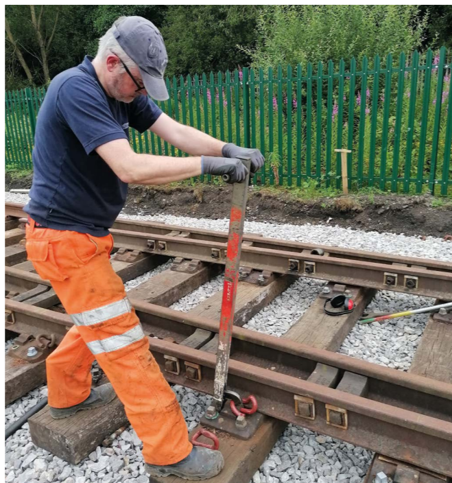
Fitting a Pandrol clip to a fishplate.
