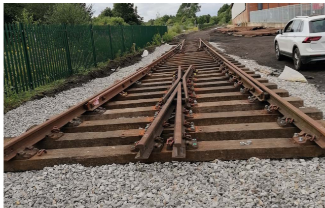
One of the new turnouts taking shape.
