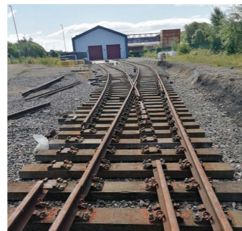
Work continues on the turnout between Otley Terrace and DLW.
