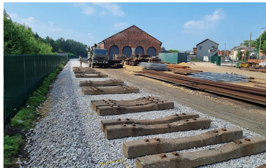
507 STRE laying out concrete sleepers in advance of main works.
