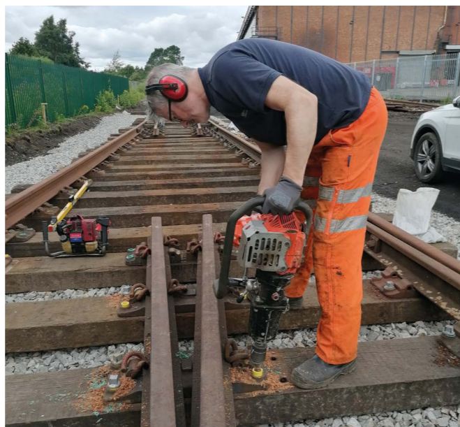
Tightening fishbolts.
