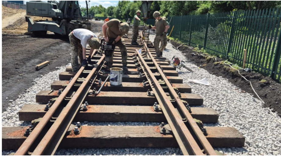
507 STRE installing a Cv9.25 turnout in early June.
