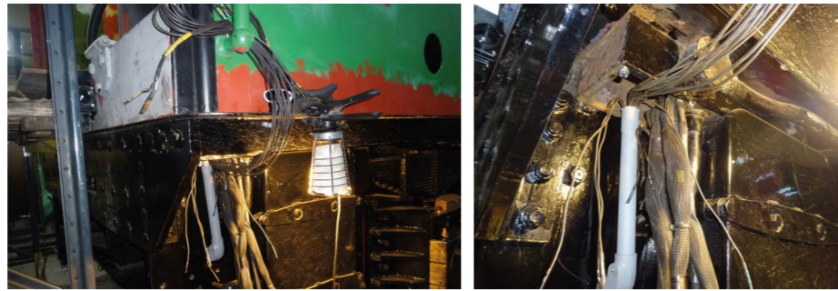
Above left: Replacement fireman's side cross-engine conduit with loom ready for re-termination.
